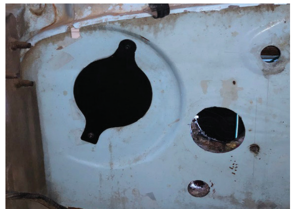
Photo 2 - Install Block-off to fire wall
