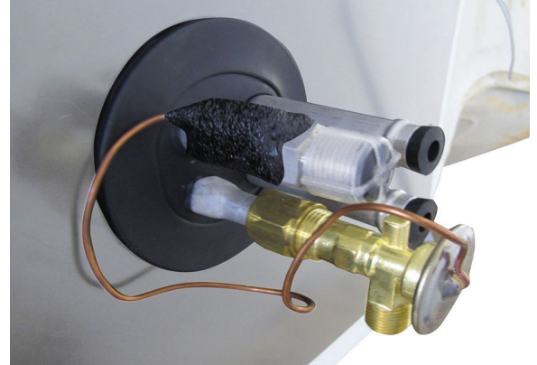
Photo 12 - Wrap Expansion Valve Sensor
