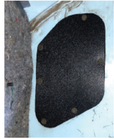
Photo 3 - Install Fresh Air Block-off plate.
