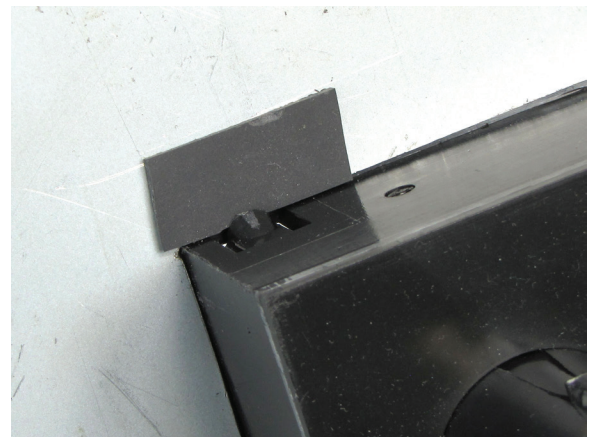
Photo 10 - Attach Adhesive Spacer Strips
